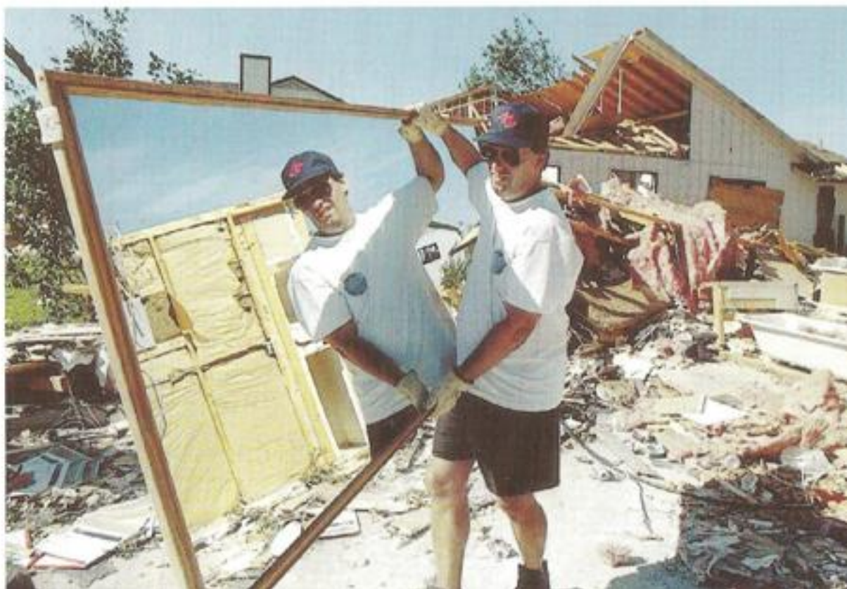
Texas: after a tornado
