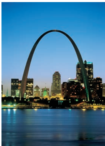
Glen Allison/Stone/Getty Images The design of the Gateway Arch near St. Louis is based on an inverted hyperbolic cosine curve (Exercise 73).
