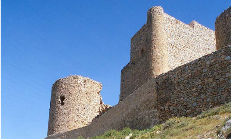
The curtain wall and turret of the outer bailey.
