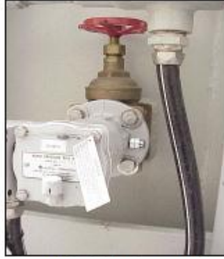
شكل 3-15 : Sudden Pressure Relay
