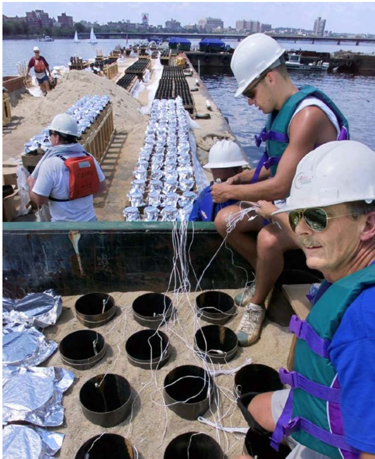
Wiring the circuit board
