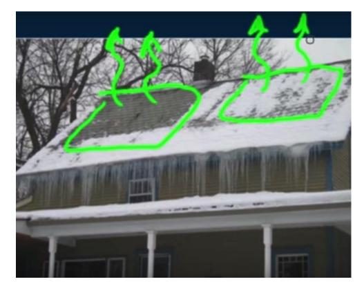
Snow patterns on the roof of a house show areas of conduction and insulation. Bare parts show where heat from inside has conducted through the roof and melted the snow.
